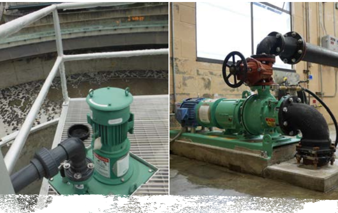
Primary Clarifier Scum
